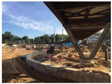
Granite walls under steel bridge over Cook Park's pond are currently being installed. When complete, park users will be able to walk in this area near the water.
